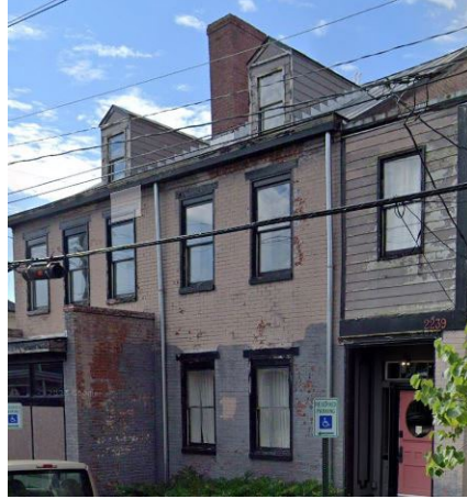
Figure 8. Example of shallowly pitched gabled roof with dormer windows on Venable Street in Union Hill.
