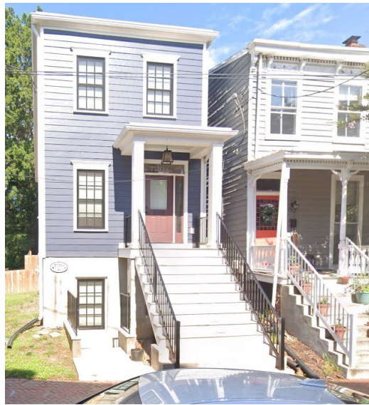
Figure 10. Example of new construction using an English basement at 720 Jessamine Street in Union Hill.
