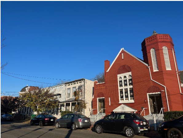
Figure 3. Looking north on Venable Street at the corner of N. 22 nd Street.
