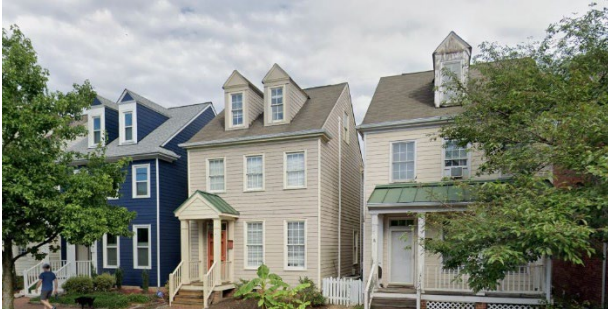
Figure 7. Examples of shallowly pitched gabled roofs with dormer windows on new construction on 500 block of N. 24 th Street in Church Hill North.
