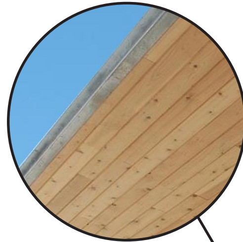
wood shiplap ceiling with break metal gutters and rain chains
