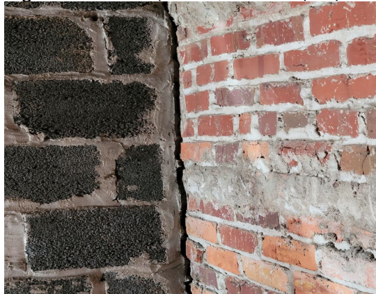
Figure 4. Wall separation and improper repairs.
