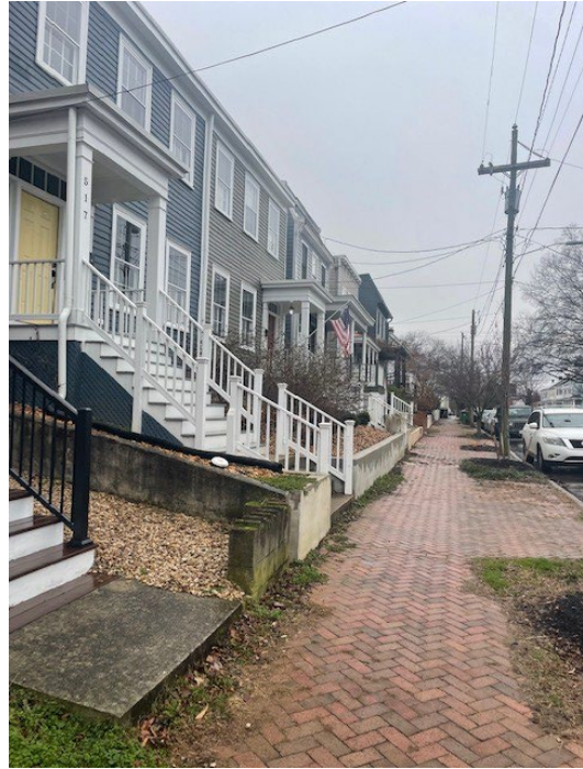
Figure 4. walls on block
