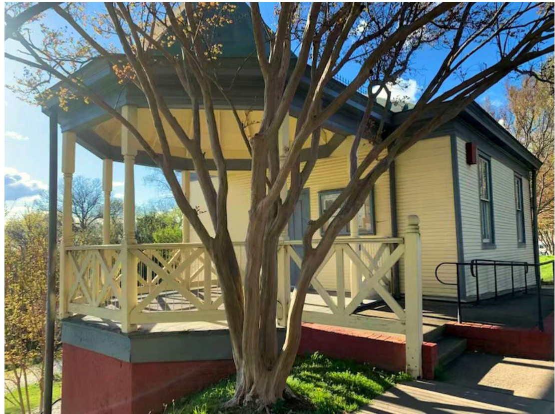
View from north east corner
