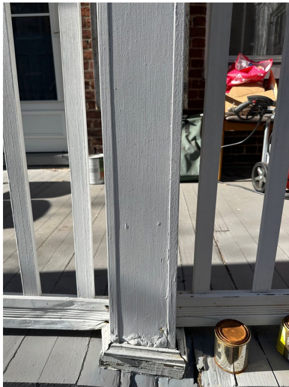
Fig 2 – Porch support beam
