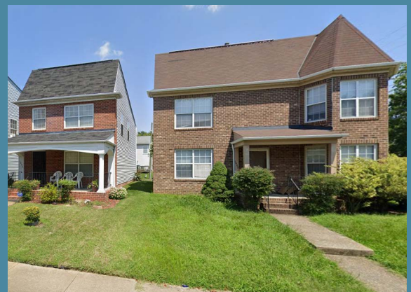
The single-family housing constructed after the leveling of Randolph.
