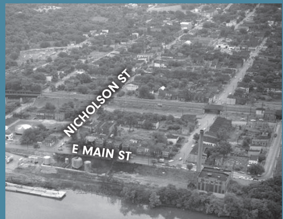
Fulton Bottom in its original urban grid pattern. The mixed-use neighborhood would be entirely leveled and replaced with suburban single-family housing.
