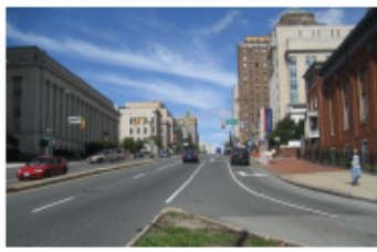
Photograph 4 - Broad Street at N. 14th Street Intersection from Southbound I-95 Off-Ramp
