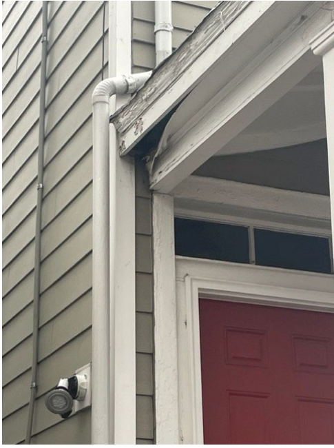
Figure 3. 509 N. 29 front porch deteriorated wooden elements.
