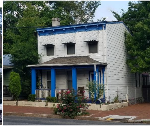
Figure 8. 422 North 26th Street.
