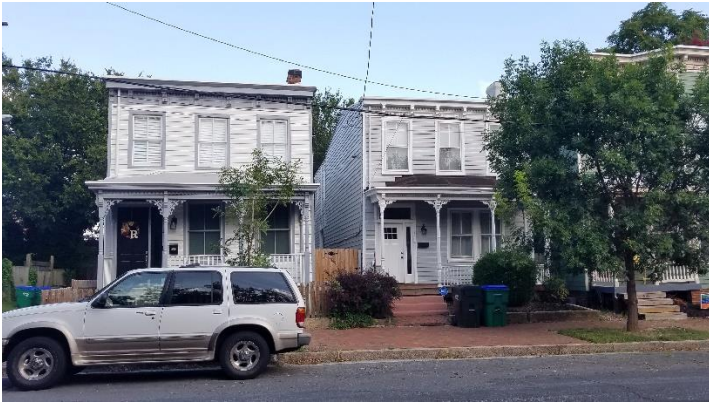
Figure 9. 412 and 414 North 26th Street.
