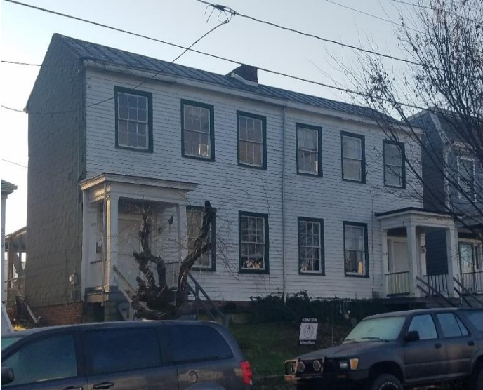
Figure 1. 515-517 North 28th Street, façade
