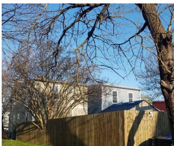
Figure 4. Rear massings on subject alley
