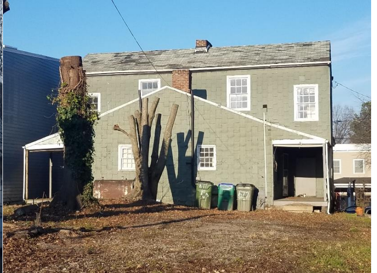
Figure 2. 515-517 North 28th Street, rear elevation
