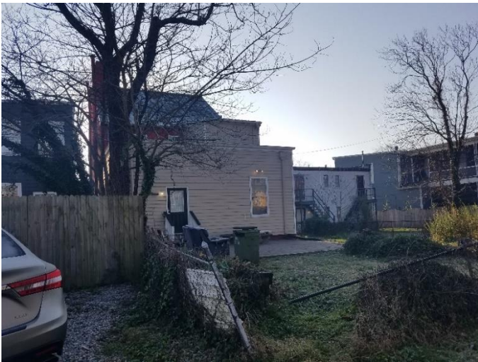
Figure 3. Rear massings on subject alley
