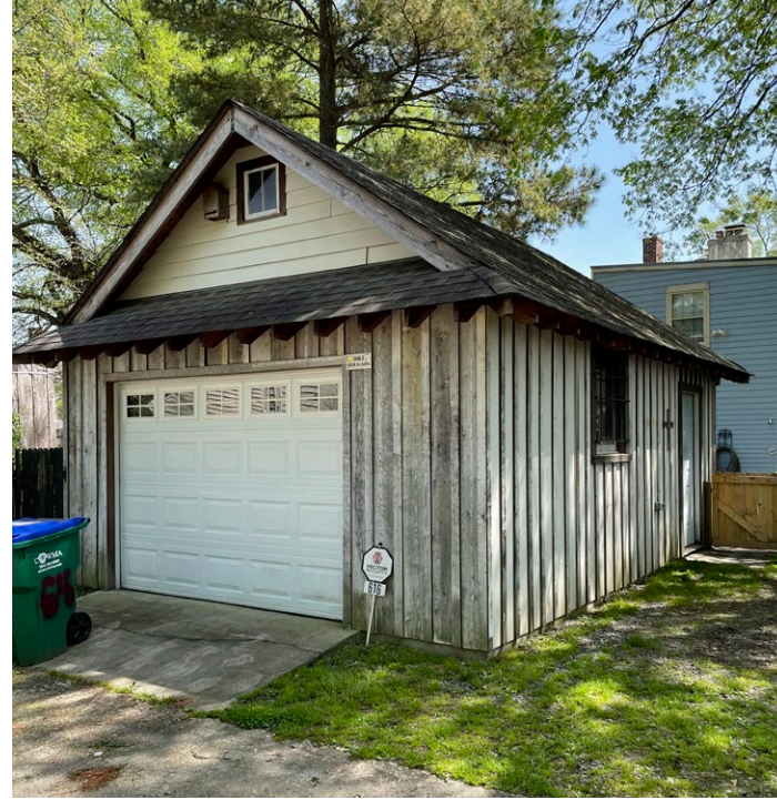
ALLEY VIEW AT GARAGE BEHIND 616 N. 27th STREET
