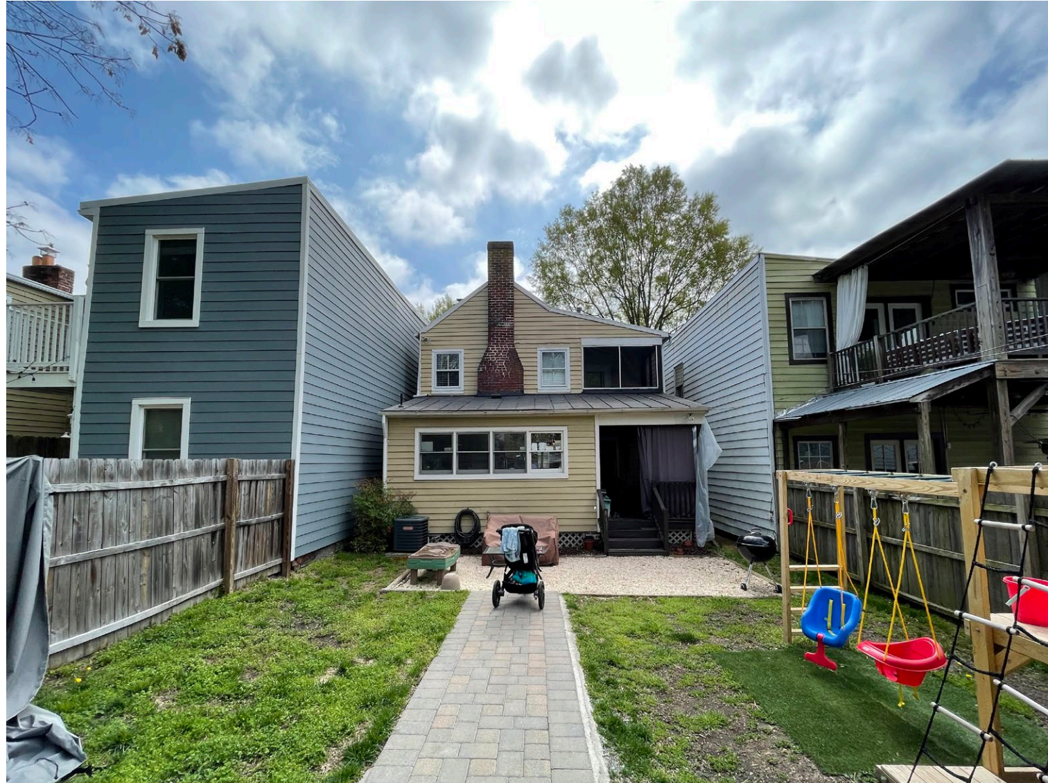
VIEW OF THE REAR WITH NON-ORIGINAL 'LEAN-TO' STYLE KITCHEN + PORCH
