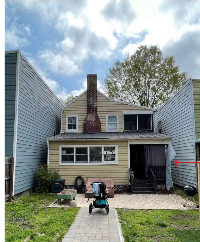
REAR OF HOUSE W/ NON-HISTORIC KITCHEN ADDITION + PORCH
