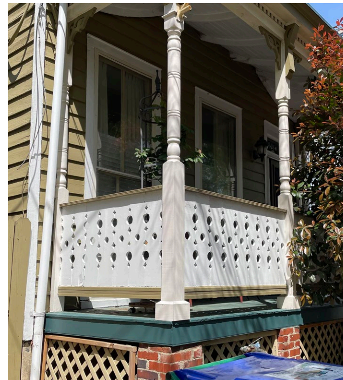
614 1/2 N. 27th STREET – DECORATIVE GEOMETRIC RAILING
