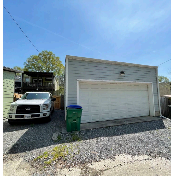
ALLEY VIEW TOWARDS GARAGE AT REAR OF 608 N. 27TH STREET
