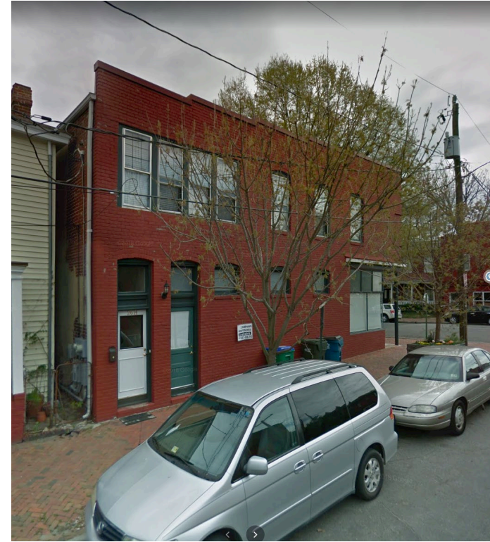
2614 E. MARSHALL ST. – WINDOW GROUPINGS ON SECONDARY FACADE
