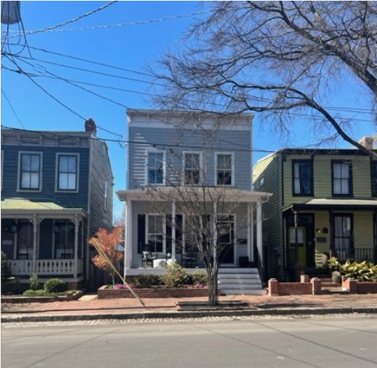
Figure 1. 608 N. 27 Front Facade
