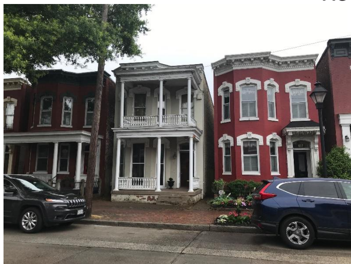
Figure 1. 415 West Clay Street, façade
