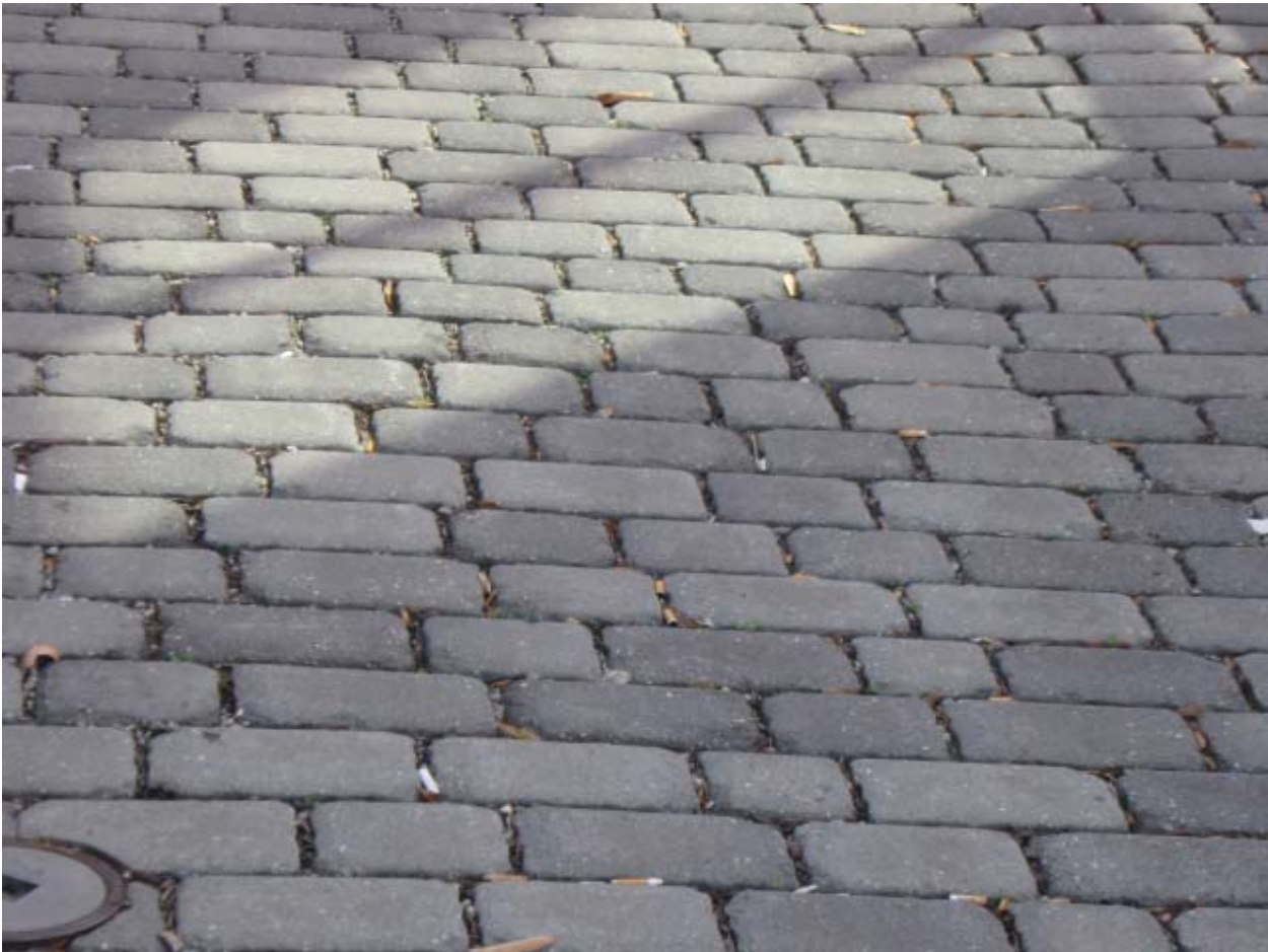
Concrete pavers used in the alley bound by E. Cary and E. Main Streets, S. 12 th and S. 13 th Streets
