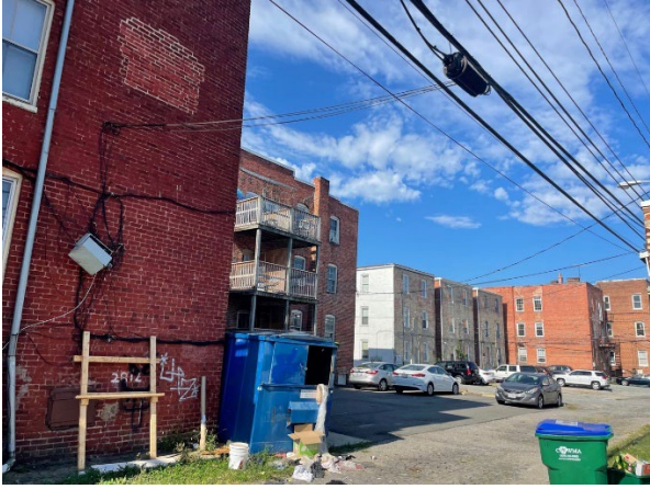
Figure 1. View of vacant lot from Monument Avenue.
