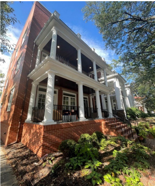
Figure 9. 2901 Monument. New constuction with substitute materials.
