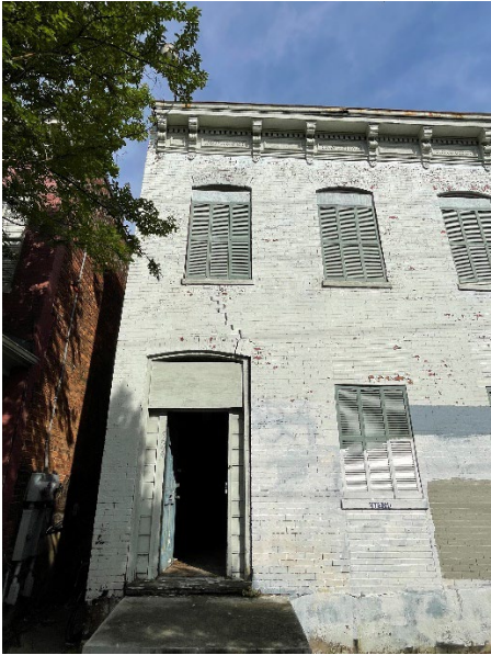
Figure 3. Separating brick on right side of façade due to failing south wall.
