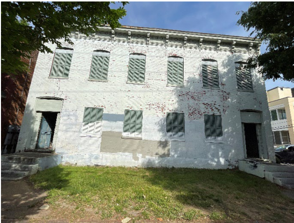
Figure 1. Façade of existing building.
