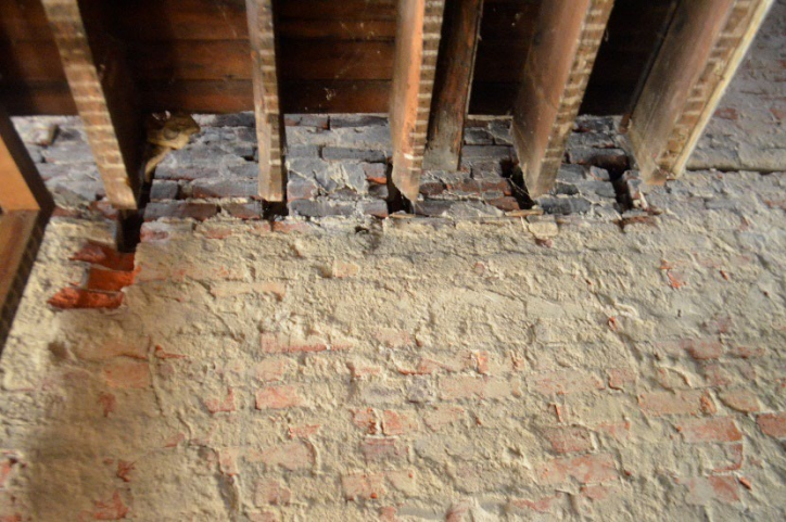
Figure 4. Floor joists separating from interior, bulging wall.
