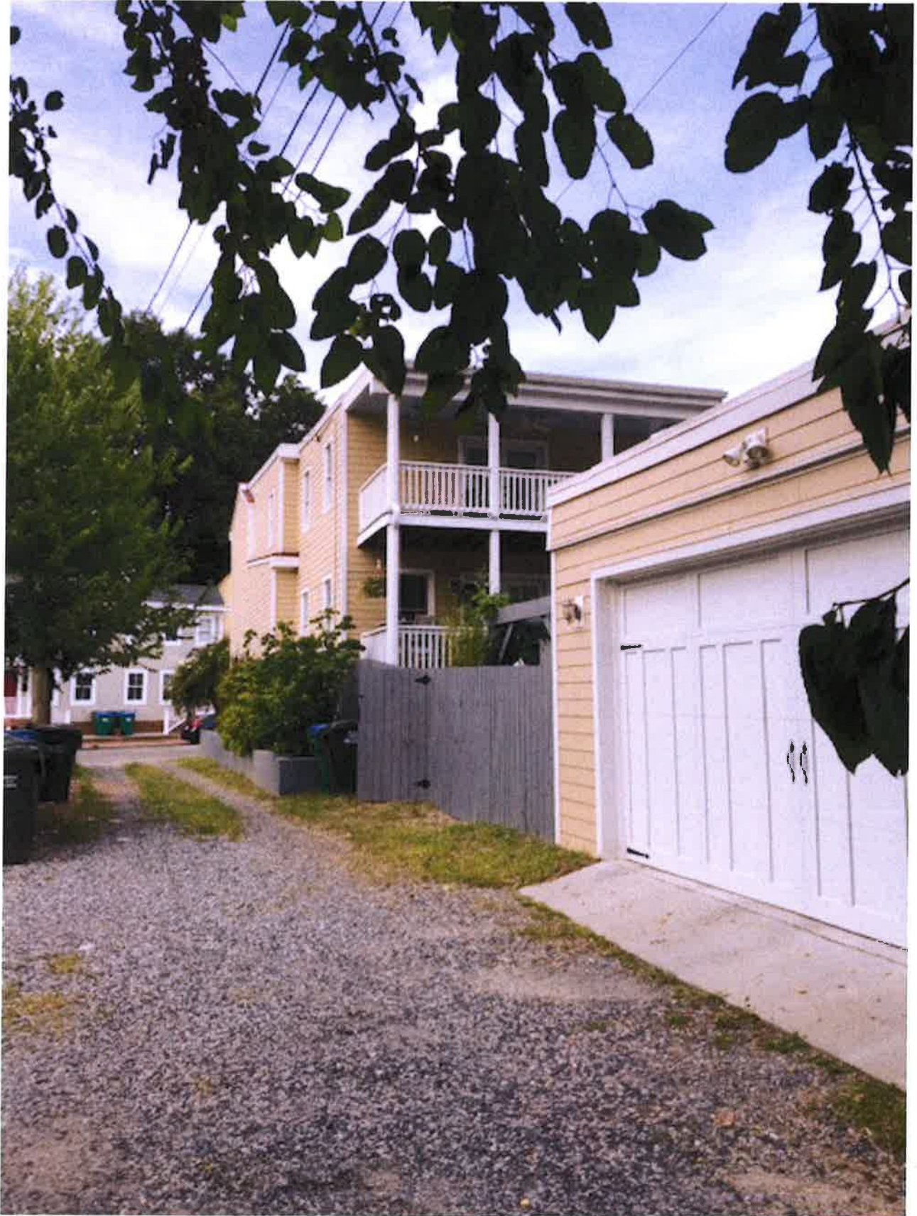
From alley looking NE toward Cedar St
