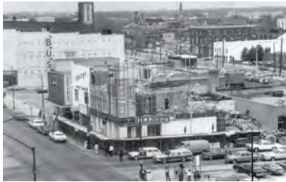
Construction of Covention Center
