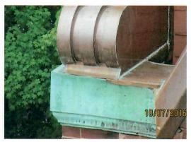
where we replaced corroded decorative details, fabricating duplicates.
