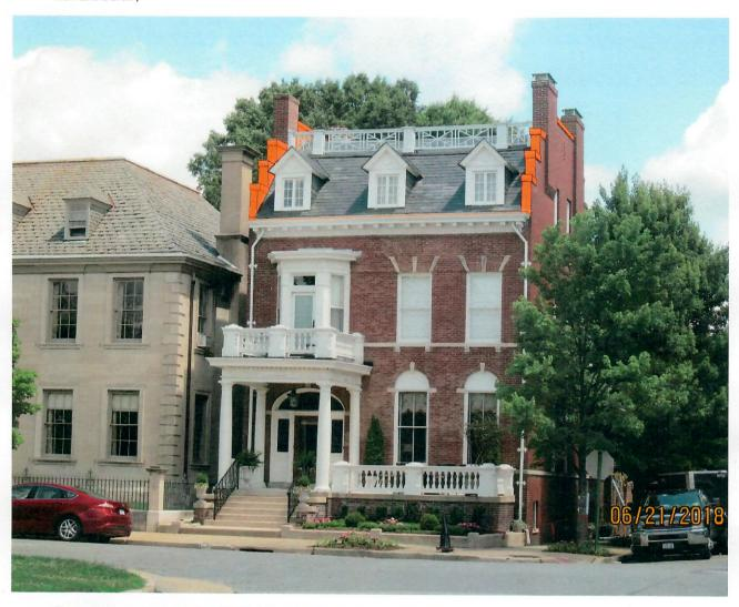
Above, is my crude rendering, using 'Paint' to illustrate ( or somewhat give an idea of ) how the front mansard parapet walls would appear with copper coping on the stepped walls. The inside faces would be covered and serve as counter flashing for the step flashing on the slate face.
