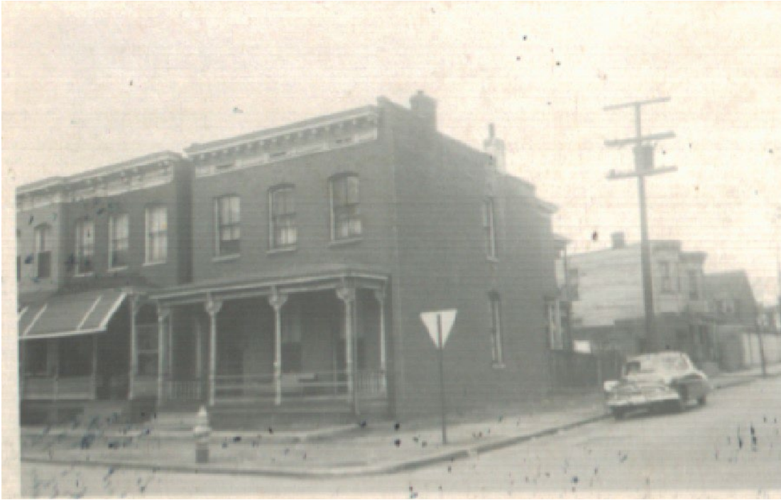
Figure 1. 1950s image of 2822 East Marshall Street. Side and rear windows are not visible in this image, or difficult to determine pane configuration due to the angle of the photograph.
