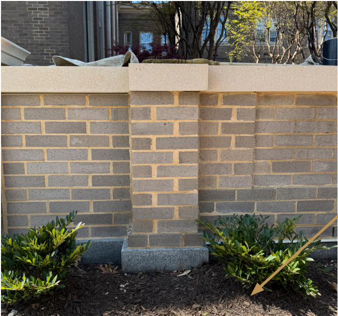
BRICK MASONRY SIGN WALL AND PRECAST PEDIMENT TO MATCH NEWLY COMPLETED RAMP WALLS
