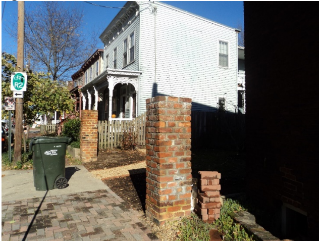
Figure 3. Brick piers in rear yard.
