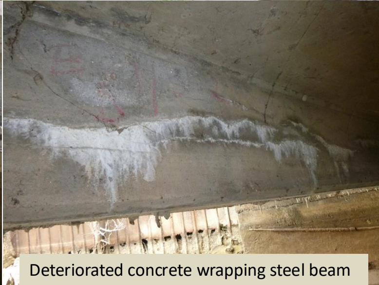
Bottom of Concrete Deck
