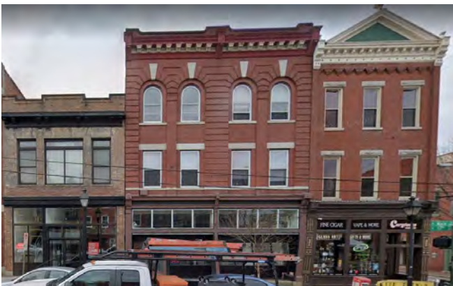
Commercial Character -- Transparent storefront and entrances at the base, a variety of window types vertically and symmetrically arranged in the middle, decorative cornices and parapet forms at the top. Subtle variations in height and color, consistent material with a variety of stone and metal decorative elements.
