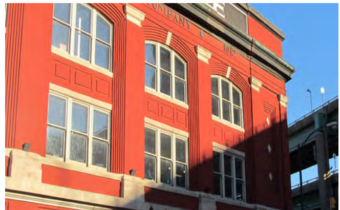
Detail -- Long facade organized vertically by pilasters and recessed wall plane containing symmetrically placed openings, decorative brickwork and stone accents.
