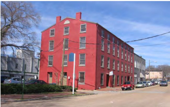
19th Century Industrial Character -- Symmetrically placed doors and windows in base, vertically and symmetrically arranged openings in the middle, and a stepped parapet at the top. Subtle variations in height, consistent color and materials.
