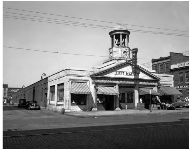
City Market, built 1913, demolished 1961 1600 E. Main Street Valentine Museum
