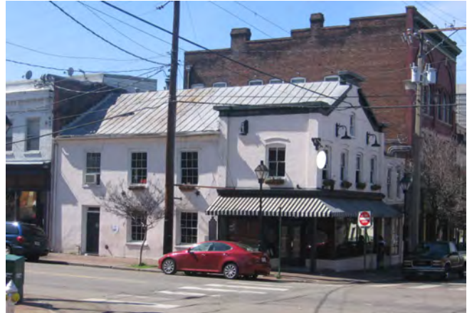
Whitlock’s Factory, built ca. 1817 1719 E. Franklin Street
