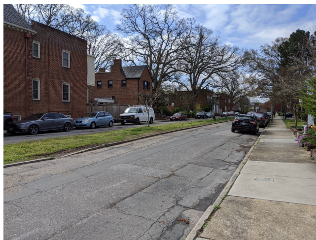
South block of Roseneath (3-24)
