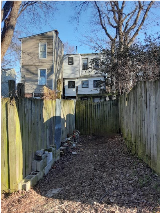
Figure 3. 412 N. 24th Street, rear elevation
