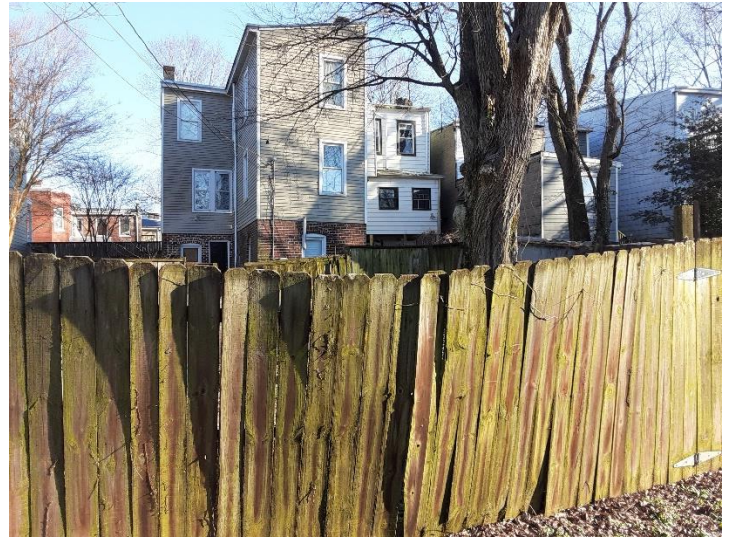
Figure 4. 412 N. 24th Street, rear elevation.
