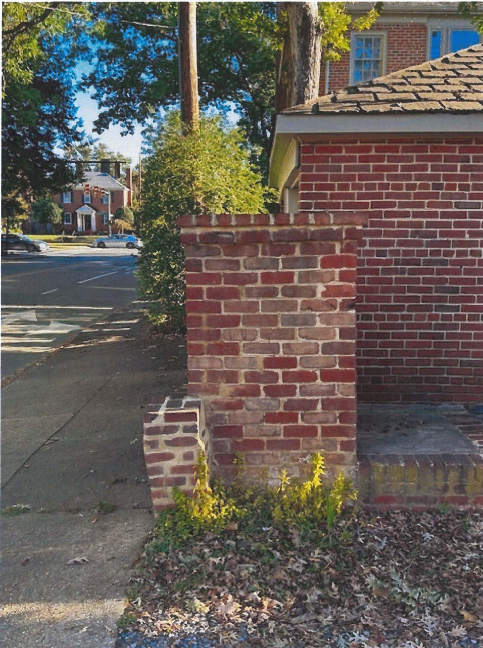
This picture shows the neighbor's garage on the rear light line with higher walls and a higher roof line.
