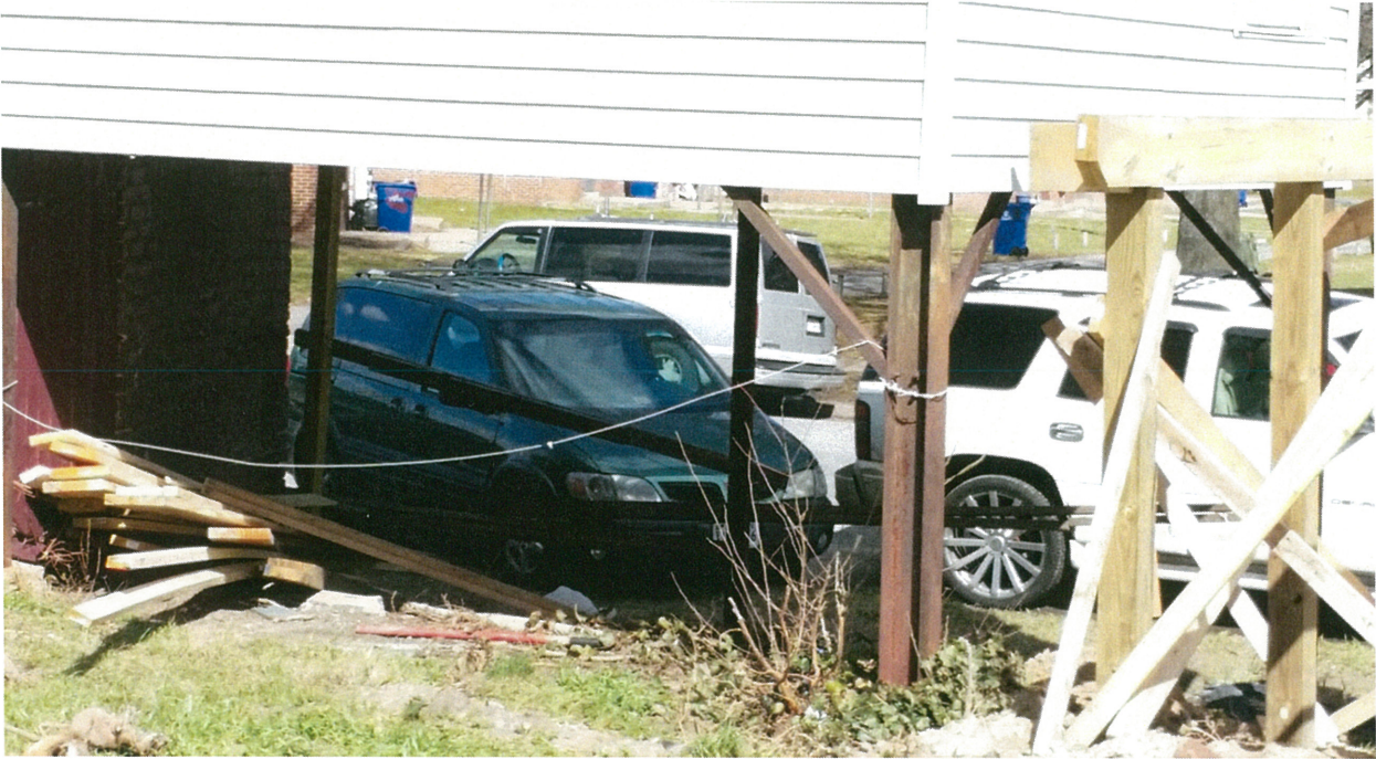
Phase "3" "Brick Off Overhang" supporting site pictures. 823 Mosby St.
