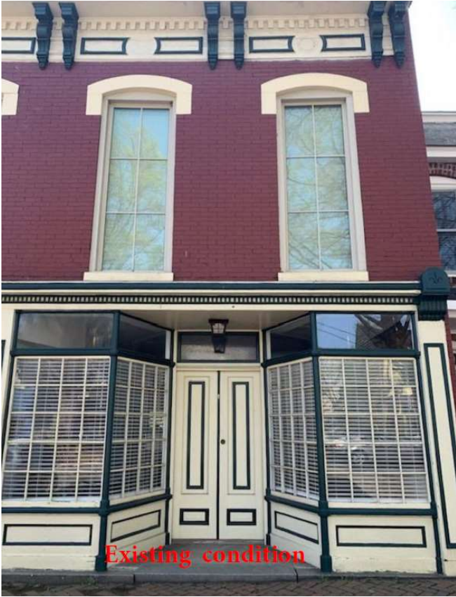
Figure 5. Existing secondary entrance with fixed doors to be replaced with a window.
