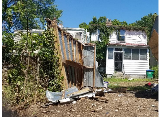
Figure 4. Remnants of shed in rear yard
