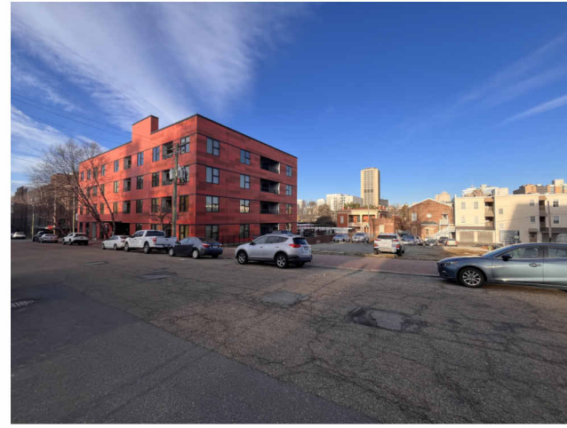
VIEW OF SITE FROM 20TH LOOKING SOUTH
