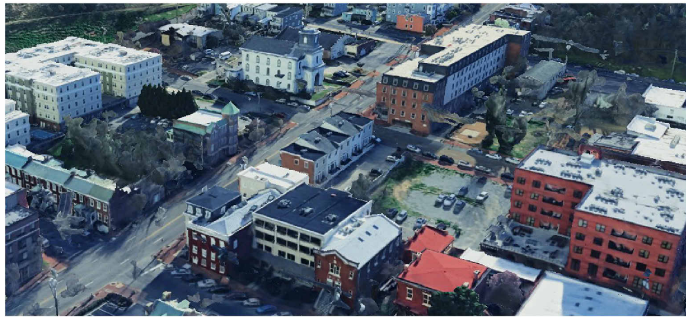
VIEW OF NORTH 19TH STREET
