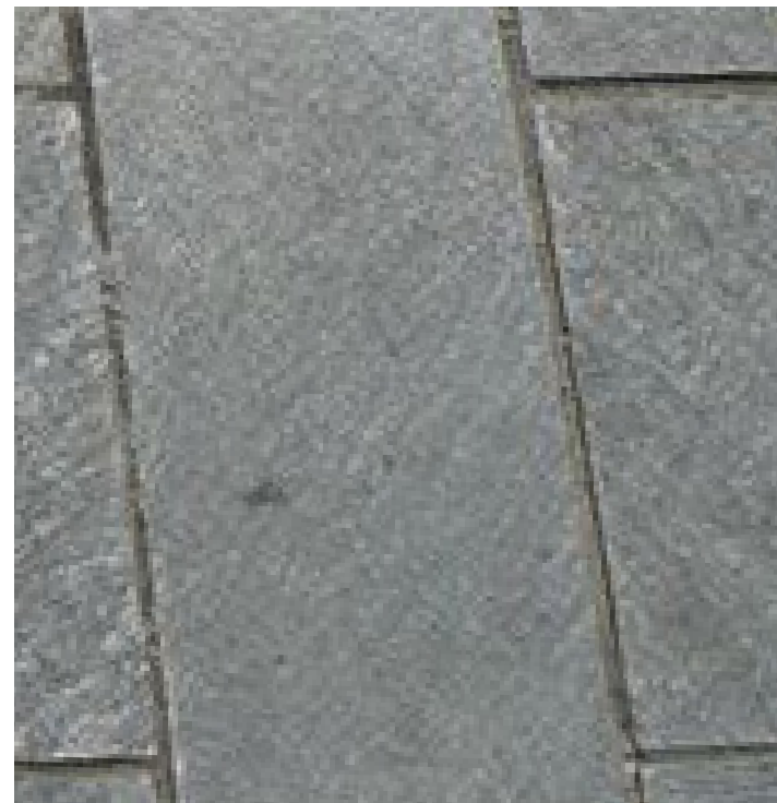
GRANITE CURBING AND BANDING
