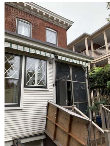
VIEW OF REAR ELEVATION TO ADJACENT PROPERTY
