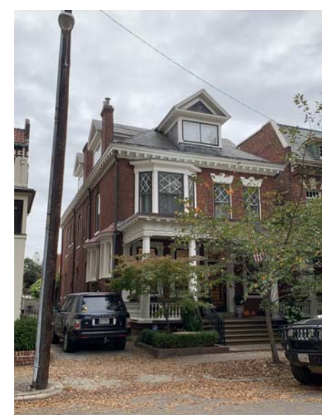
VIEW OF FRONT ELEVATION FROM N. ALLEN AVENUE
