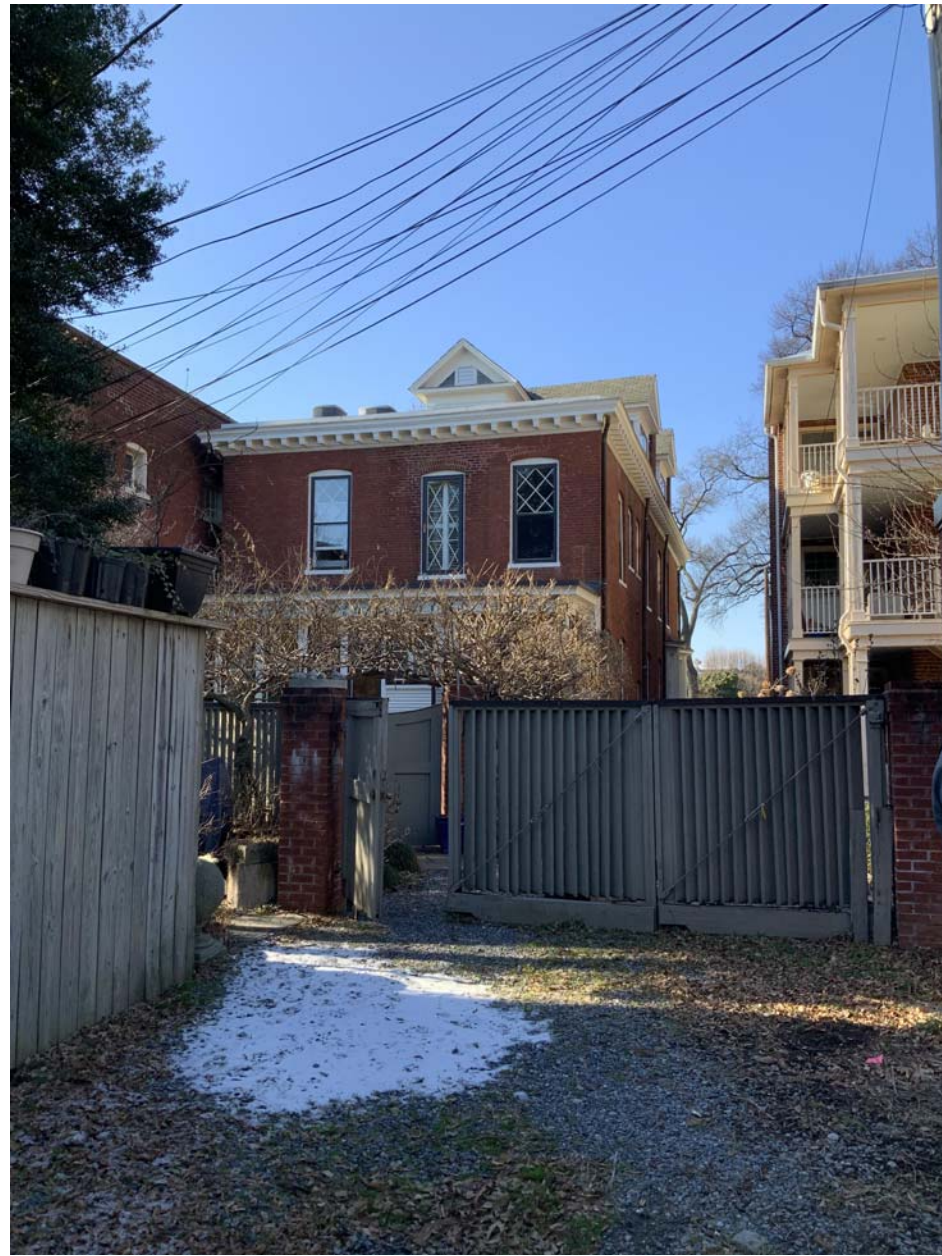
VIEW OF REAR ELEVATION FROM BACK ALLEY
