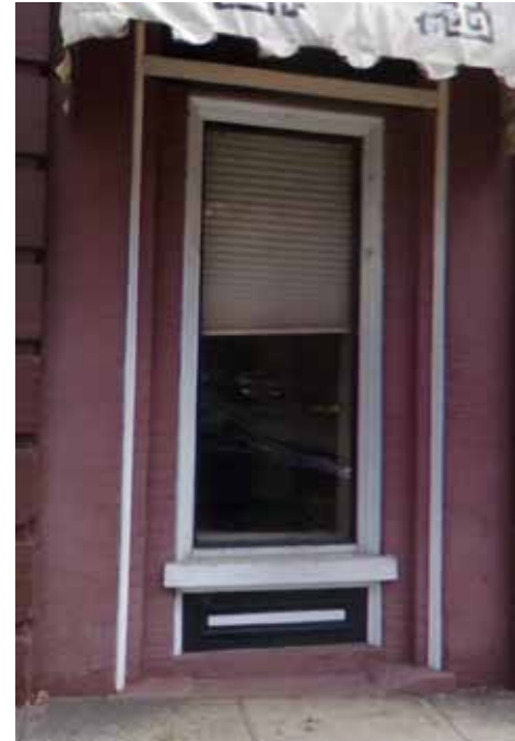
EXISTING OPENING ON GRADE
