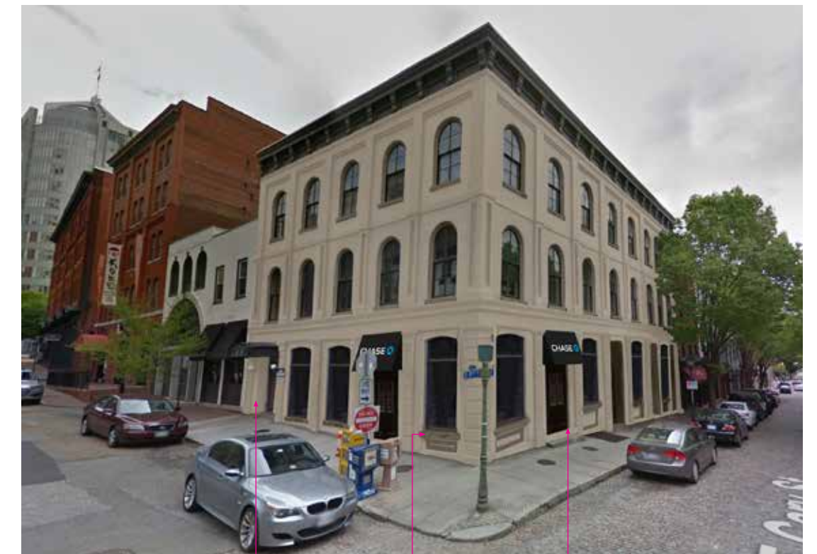
ALL BRICK - SW 7045 ALL WINDOW AND DOOR FRAMES - SW 7046 ALL WINDOW SASHES AND DOORS - SW 7048
