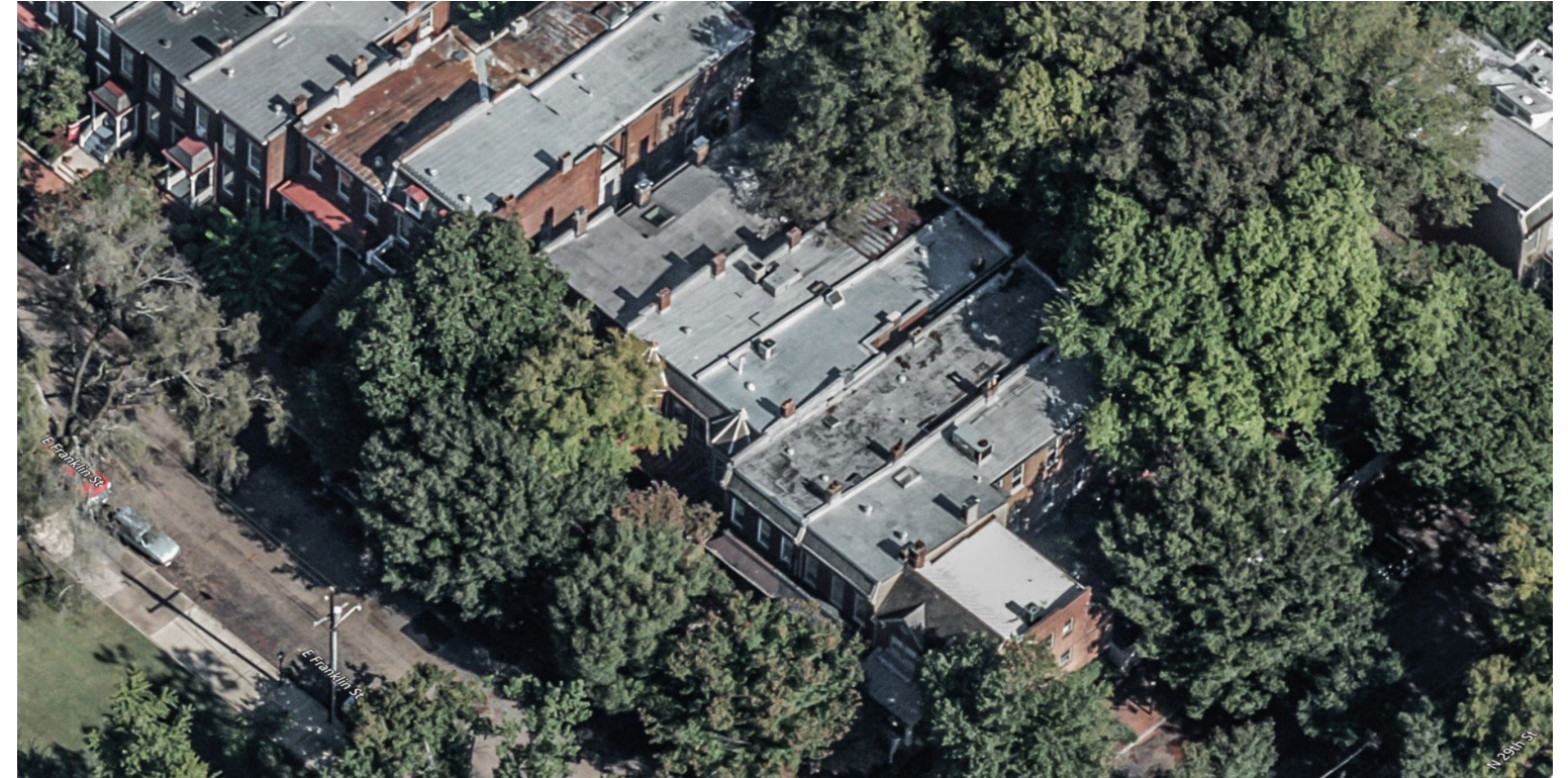
Aerial of conditions at property above E Franklin Street
