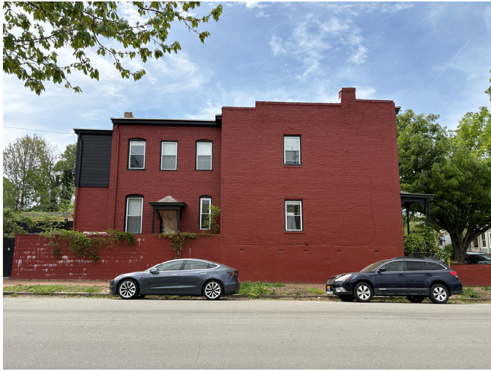
Photo-13. 427 N 26 St
