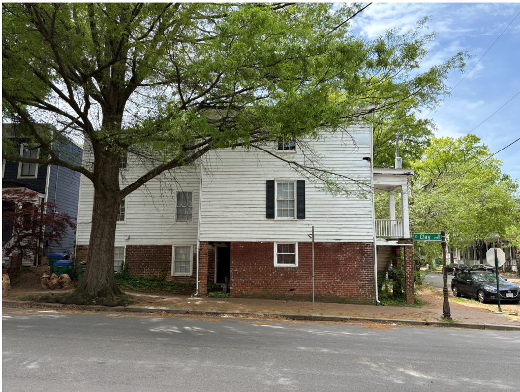
Photo-12. 419 N 27 St
