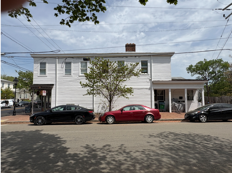
Photo-15. 501 N 25 St
