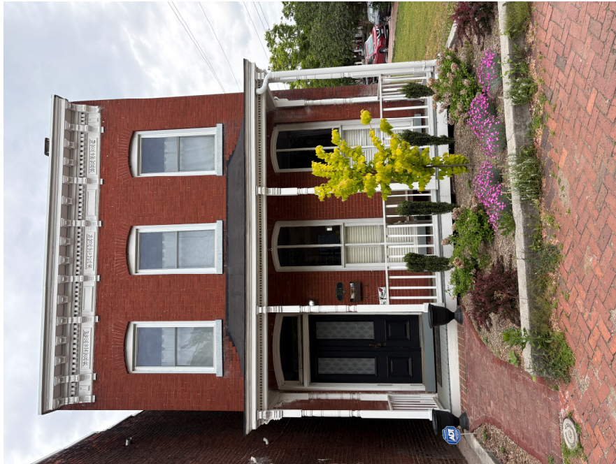
Photo-5. 2514 E Marshall St
