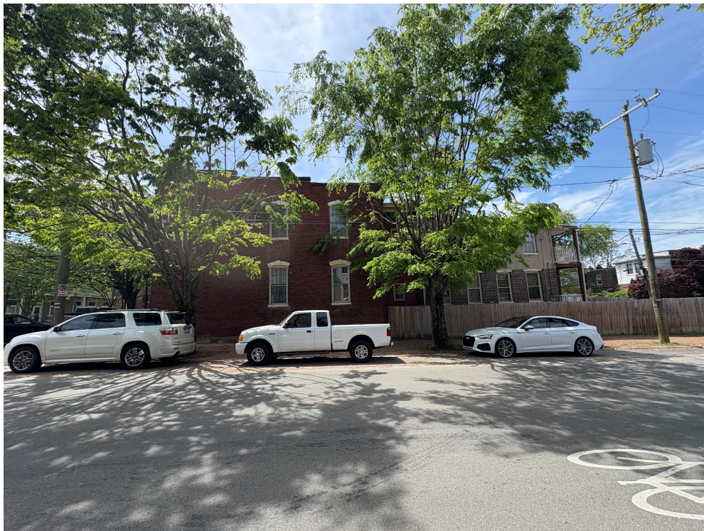
Photo-20. 324 N 24 St
