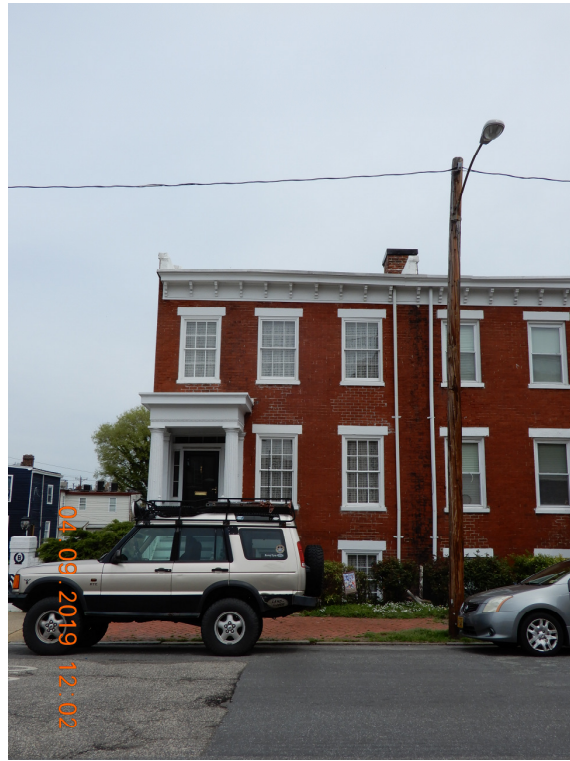
Photo-1. 2506 E Marshall St
