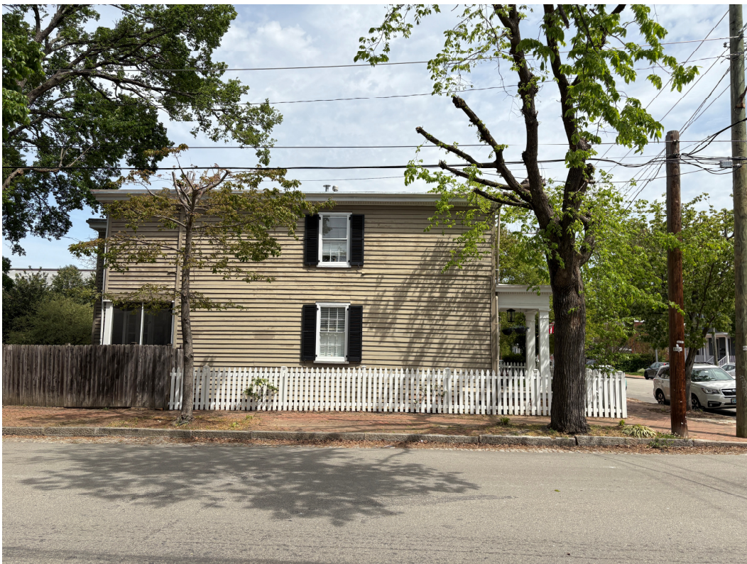
Photo-14. 500 N 26 St
