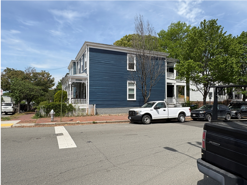
Photo-17. 2220 E Marshall St
