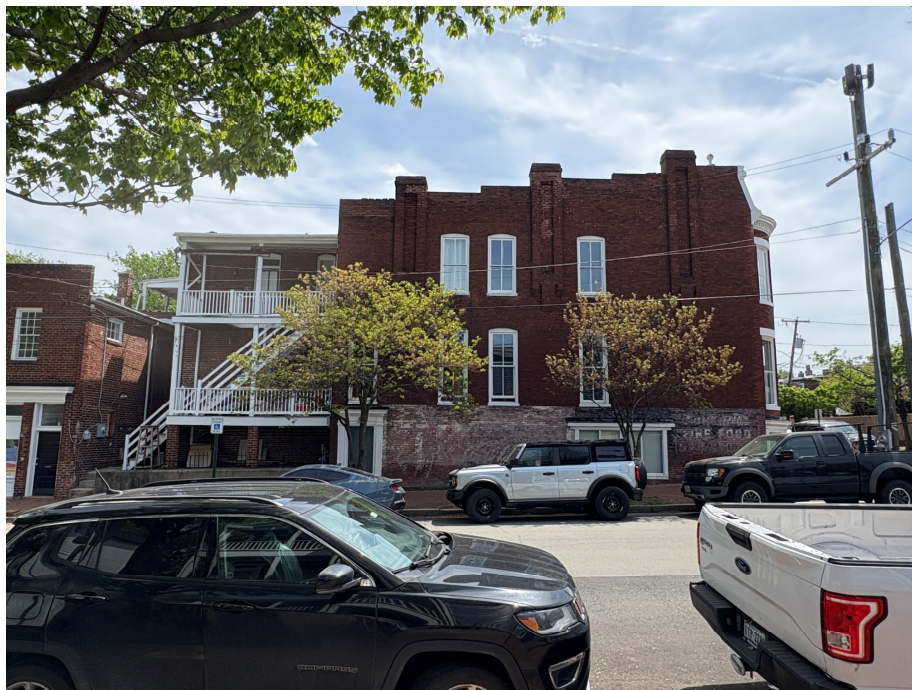
Photo-16. 2300 E Marshall St
