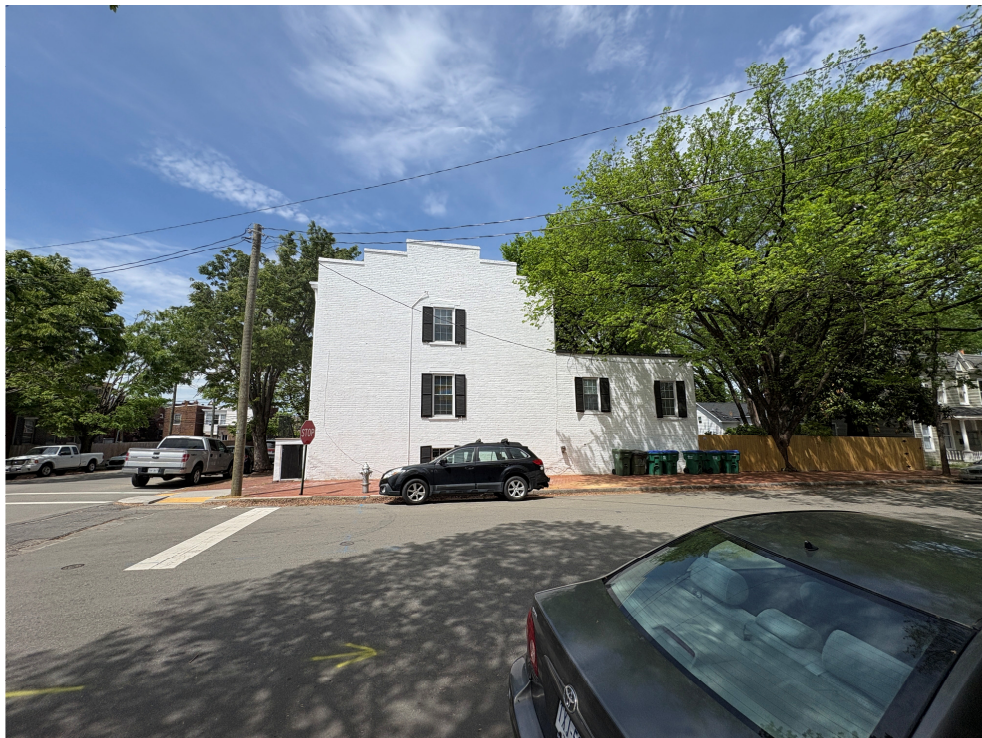
Photo-18. 2324 E Marshall St
