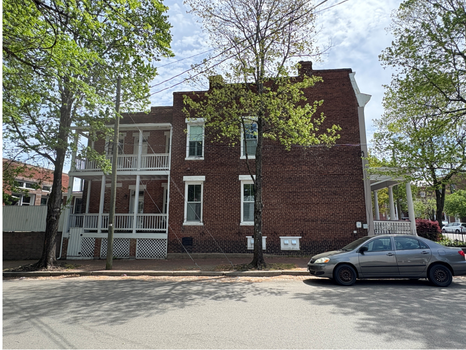
Photo-19. 2400 E Marshall St
