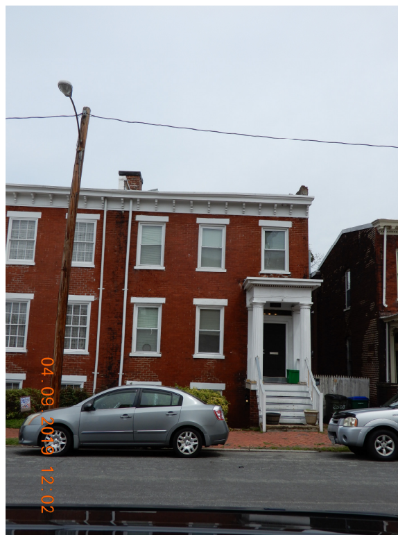
Photo-2. 2508 E Marshall St
