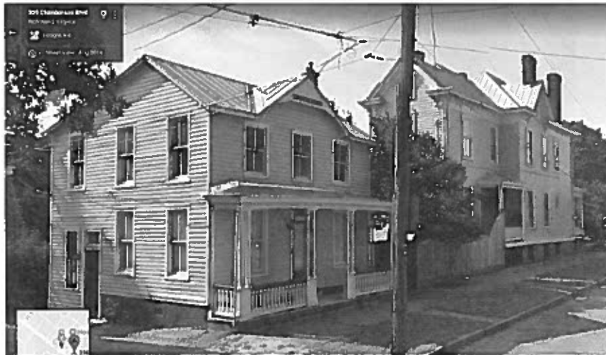
3400 E Broad Street: Two-story guest house
