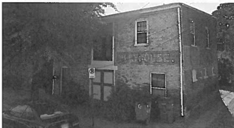
3301 E Marshall Street: Two-story carriage house
