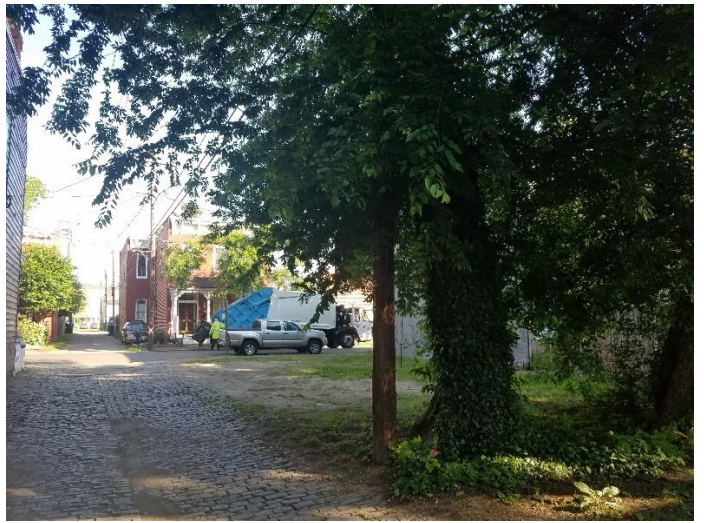
Figure 2. 521 St. James Street
