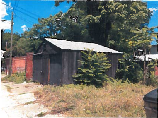
SHED ON ALLEY BETWEEN 36TH ST. AND 35TH ST.
