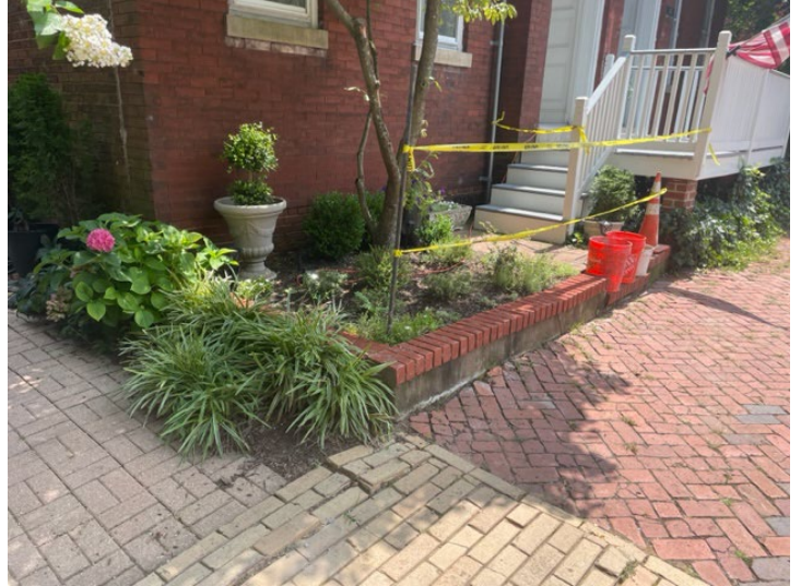
Figure 2. Staff observed work being completed without a COA on July 26, 2023. Staff sent an application page and a courtesy email to the property contact on file, suggesting they stop work and apply for a COA.
