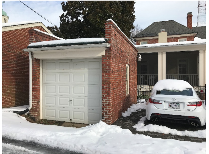
Figure 2. Garage at 3317 Monument Ave
