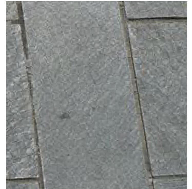
GRANITE CURBING AND BANDING
