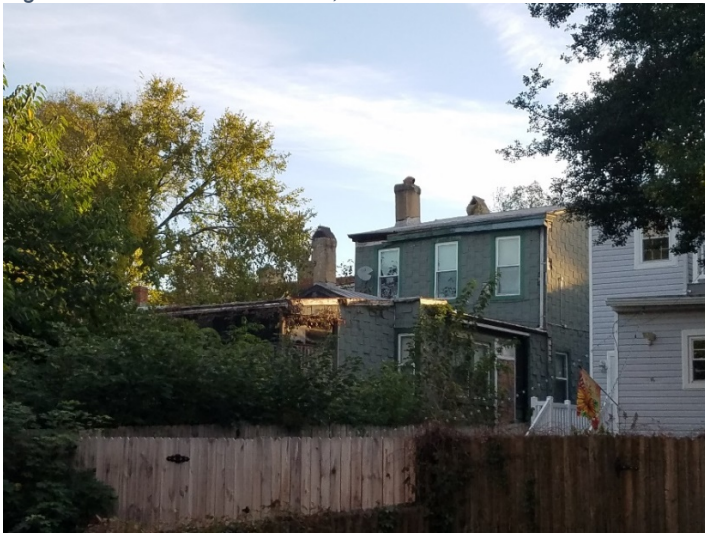
Figure 7. 706 North 21st Street, rear elevation.
