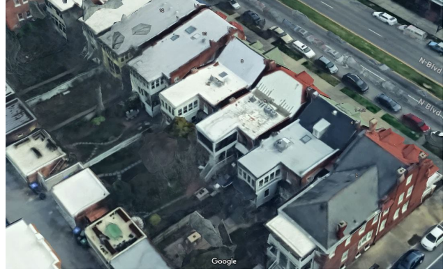
Figure 6. Arial view of clipped gable and rear flat roof.
