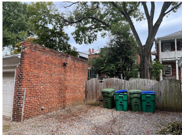
Figure 2. View from rear alley.
