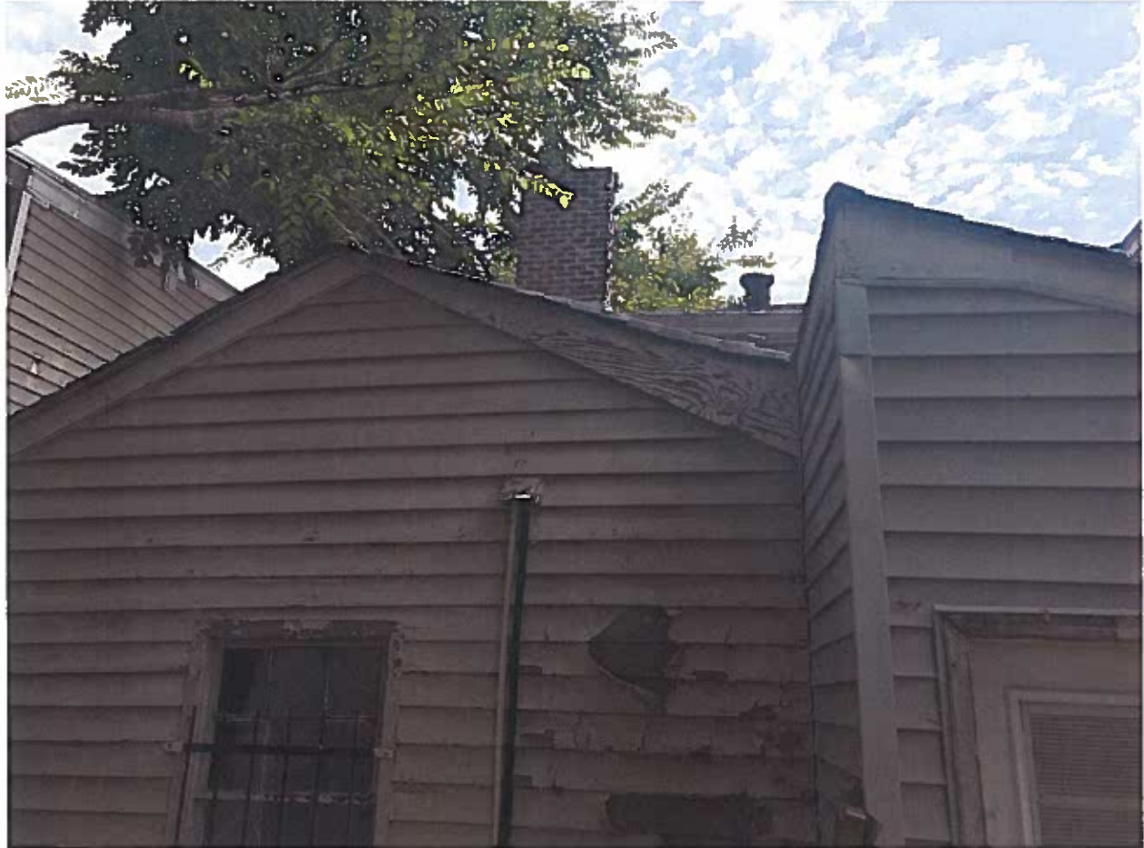
Rear Exterior showing existing asphalt shingles
