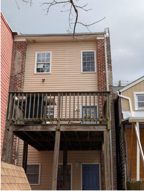
Figure 1. Existing Conditions, photo provided by applicant.
