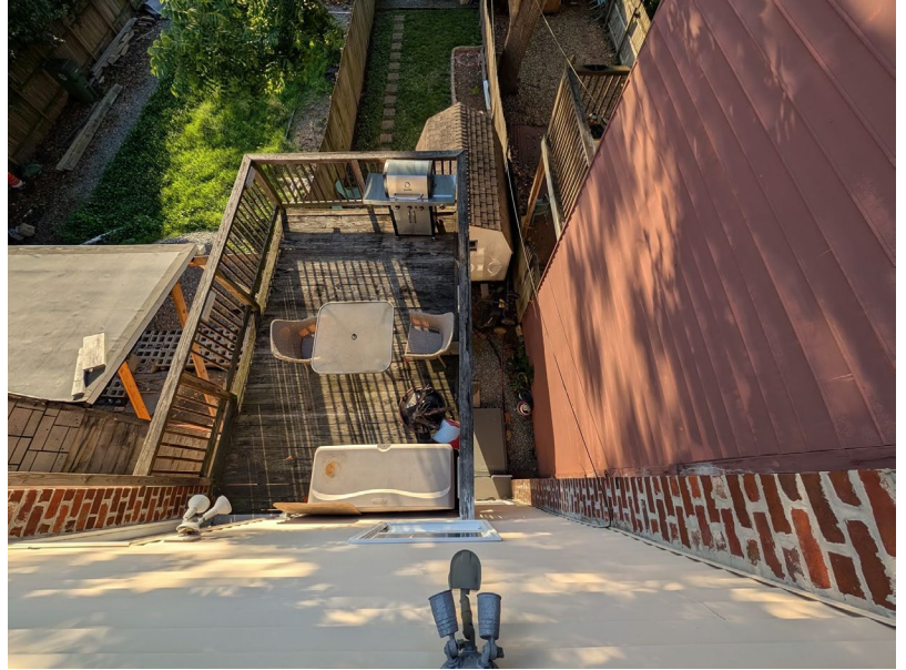
Figure 2. Existing Conditions, photo provided by applicant.
