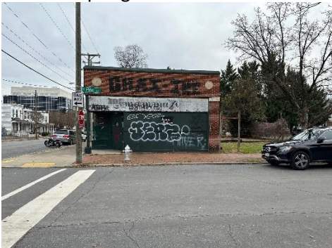
Fire Hydrant 8' in front of the existing building.
