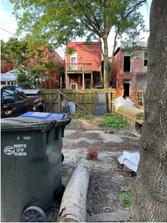
Figure 3. 3106 E. Broad Street. Existing Conditions of the rear elevation and yard.
