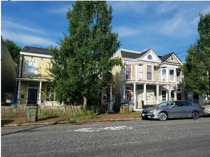
Figure 3. 33013-3015 and 3011 East Marshall Street.
